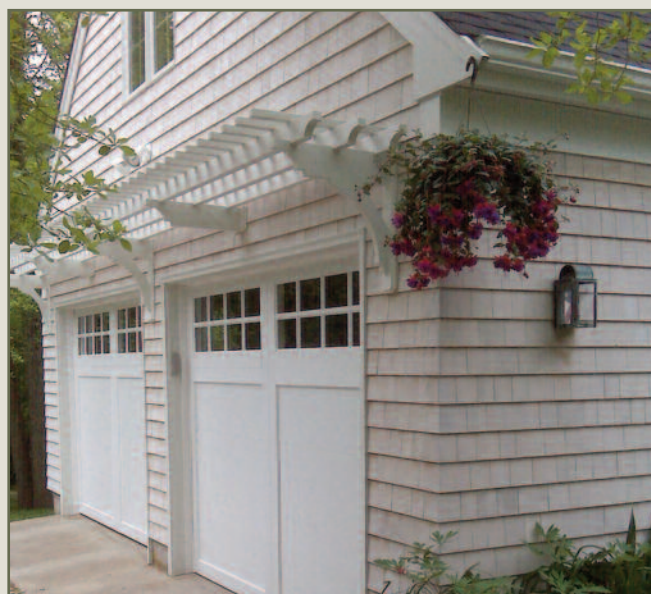
Garage Arbor Installation with Original Style
